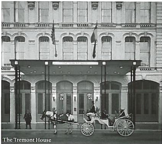
The Tremont House
